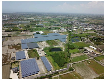
5MW Davis | Yunlin Kouhu Power Plant
